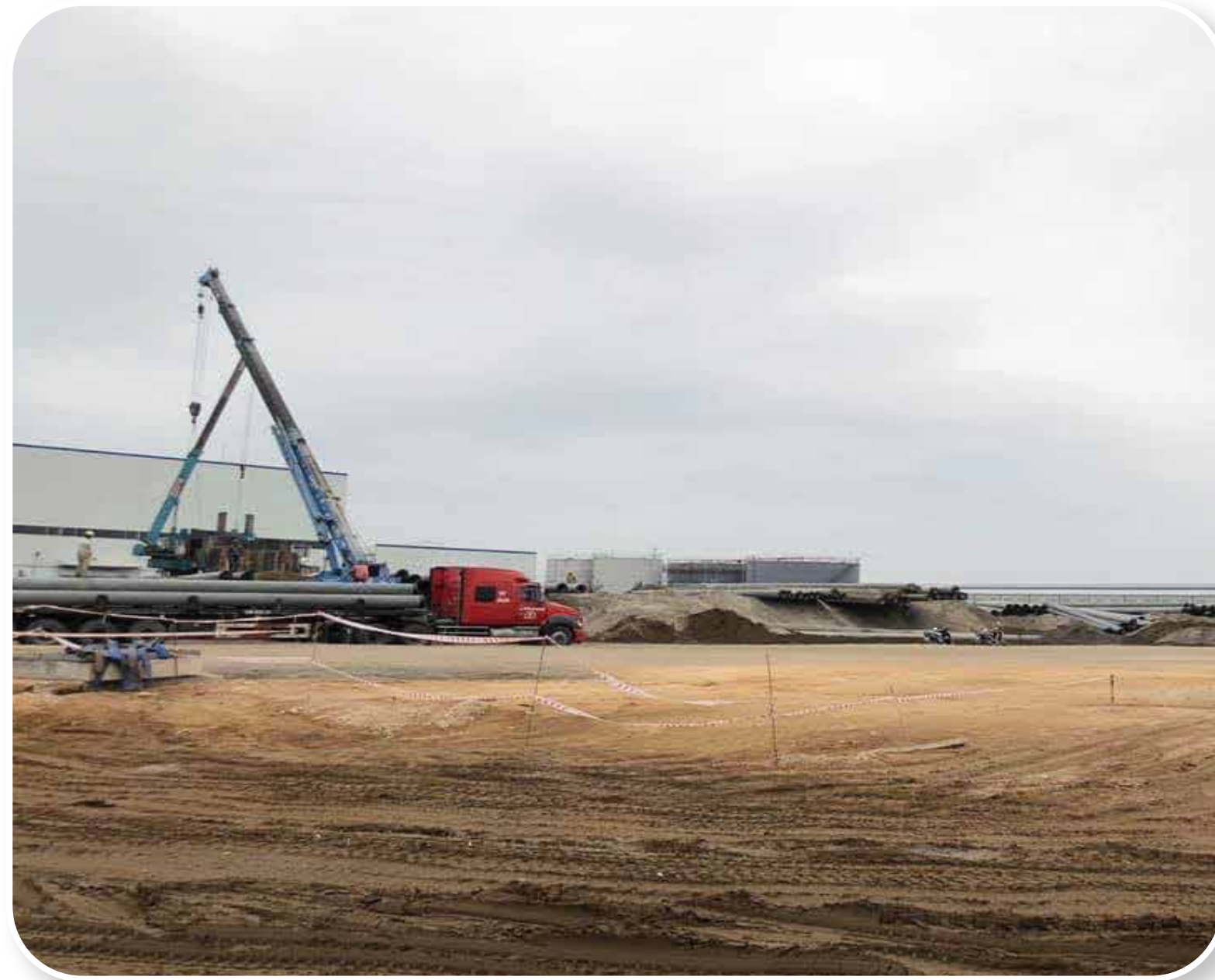
View of CFS Phase 2 construction site of Pan Hai An 2 CFS warehouses with the scale of 1 ha per each - reached the record of the largest CFS warehouse in Vietnam up to now
