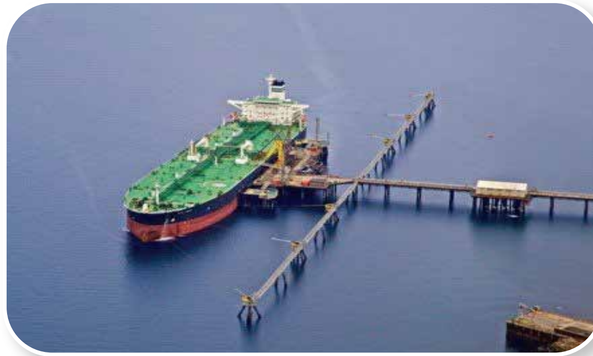
Kick off the construction of Liquid Jetty, expected to put into operation by early 2021
