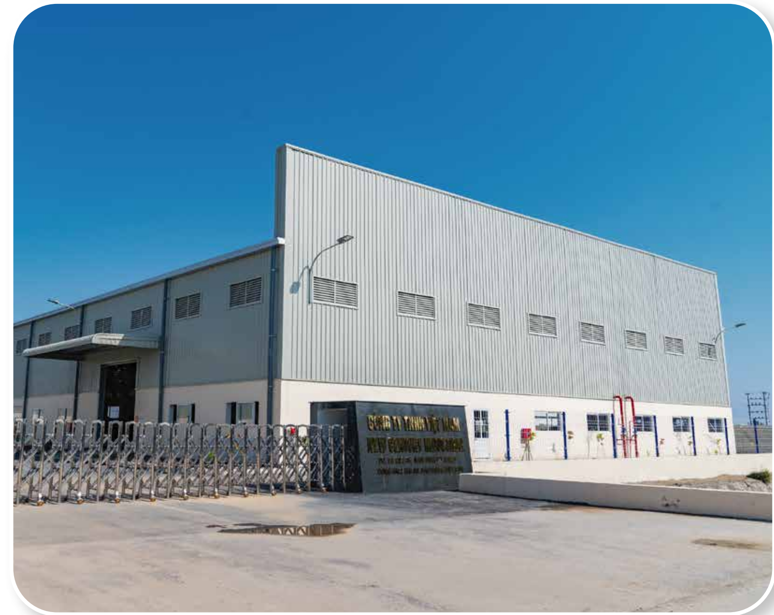
Ready Built Factory in Nam Dinh Vu IP was already handed over to customers and is in stable operation at the moment
