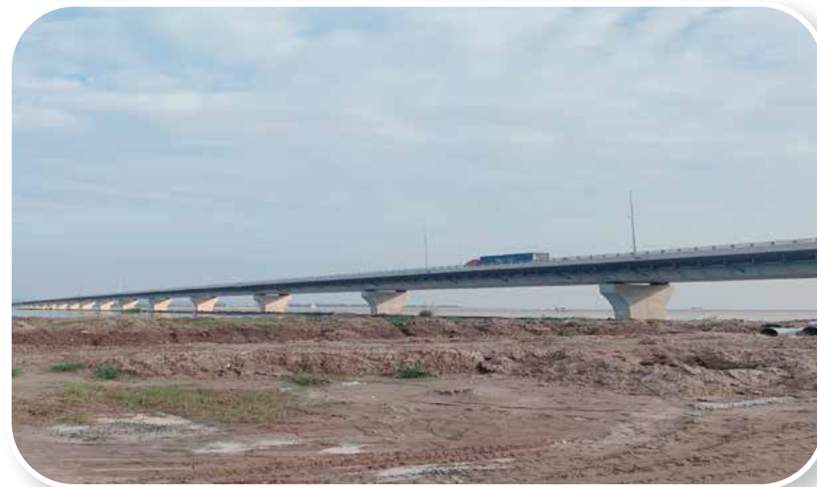
Phase 2 of Nam Dinh Vu IP is currently in the process of filling 50% of the site, and is expected to hand over 210 ha with infrastructure by June 2020
