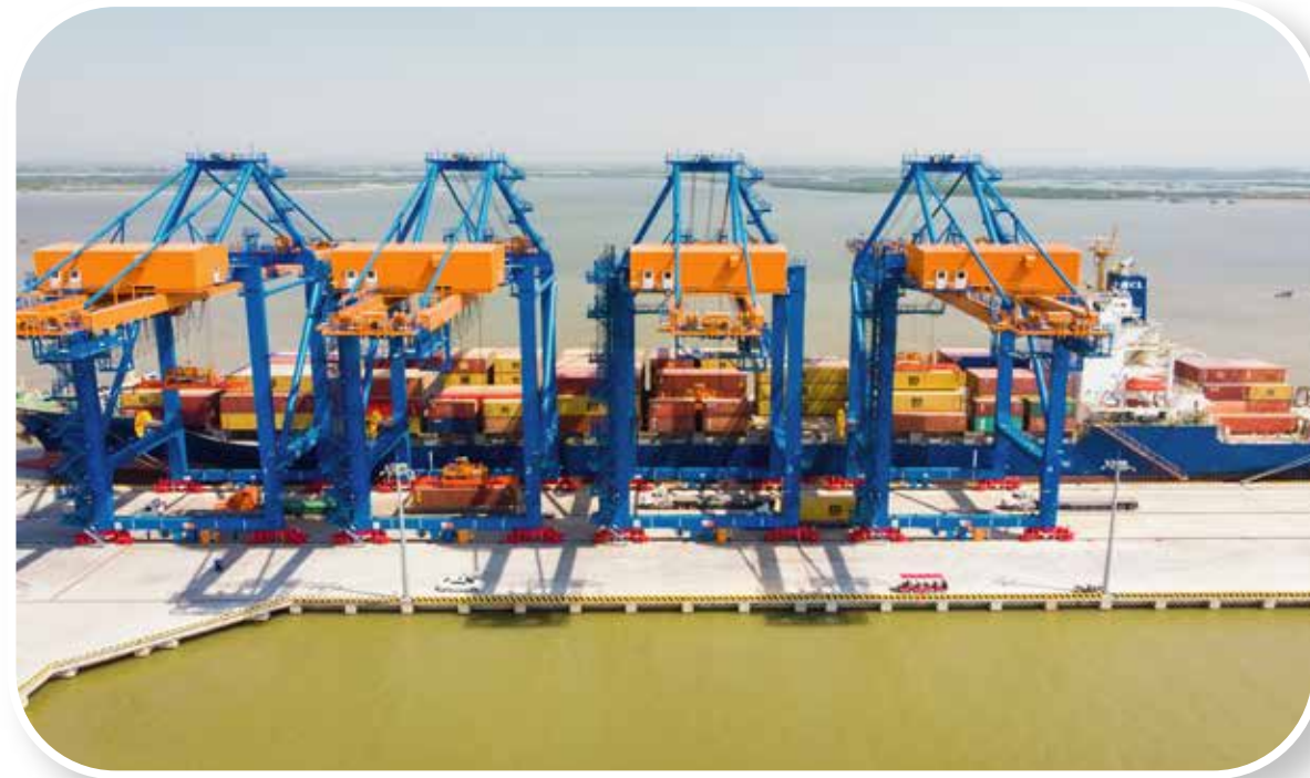
Phase 2 of Nam Dinh Vu Sea Port has been investing with the total exploitation capacity of 2019 being 150% compared to 2018
