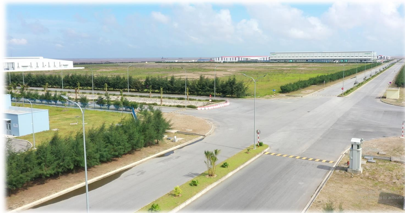
The landscape and infrastructure of Phase 2 have been prioritized for continuous investment and upgrading.
