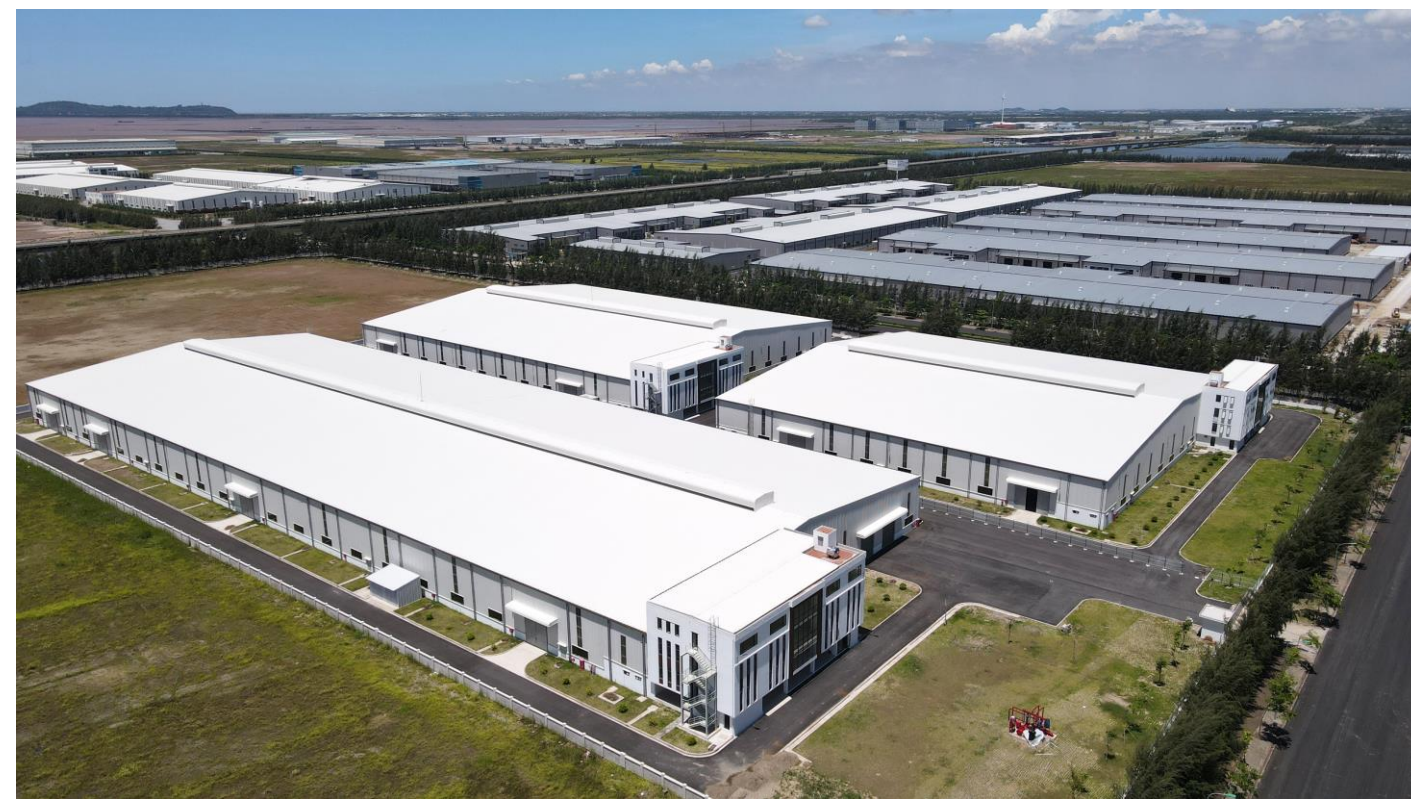
The Tuong Vien Nam Dinh Vu expansion project has been completed and is ready for operation
