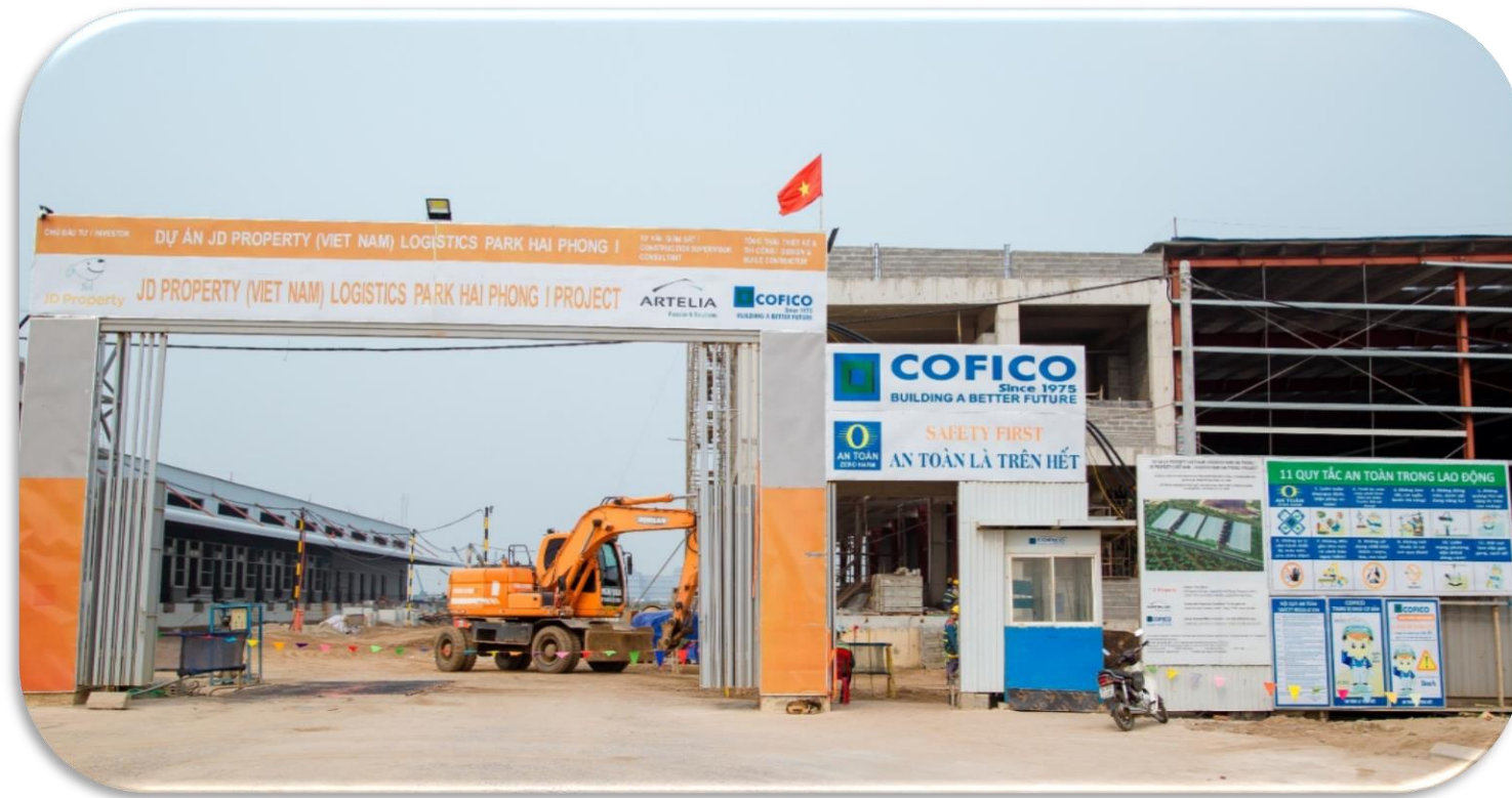
1 corner of the JD Property project site
