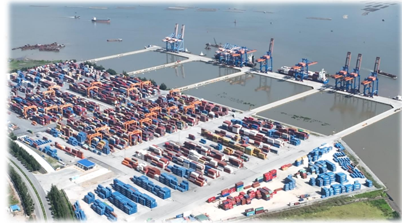
The current scenery of Nam Dinh Vu Port after being officially put into operation in Phase 2
