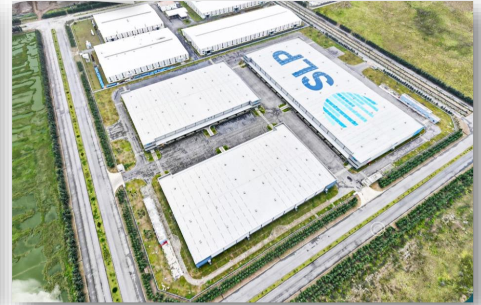
SLP Park - a smart warehouse project with optimized space
