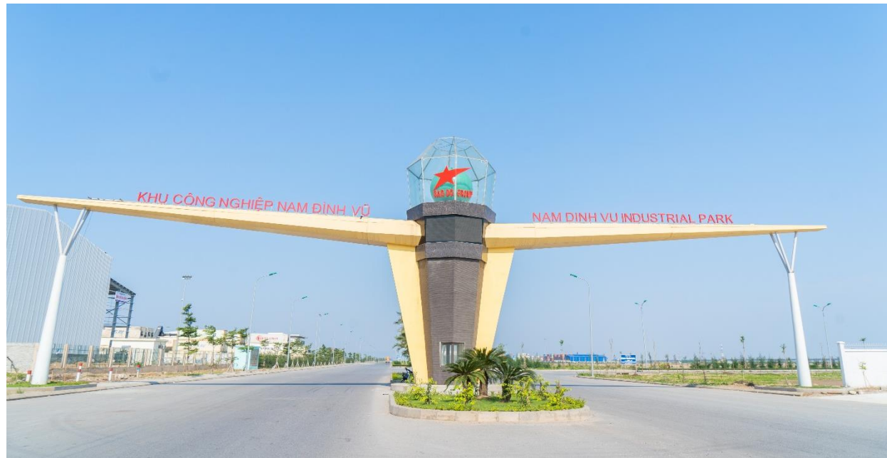
The main gate of the Industrial Park has been “uploaded”
